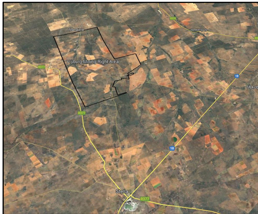
Figure 3: View of the roads that will be used to access the proposed mining area (image obtained from Google Earth).
